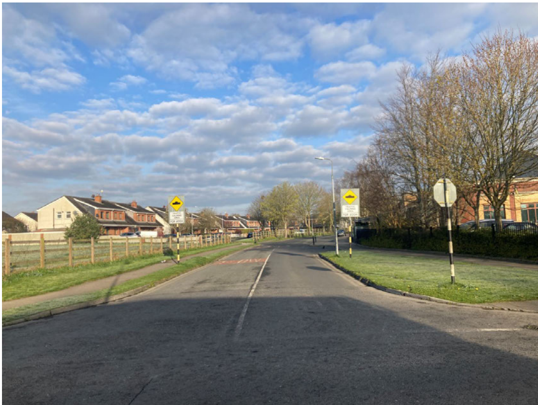
Image 2 – Traffic Calming Signs on Beaufield Road from Meadowbrook Road End
